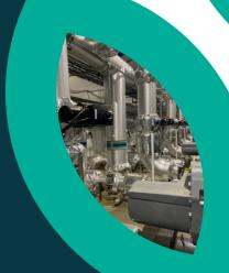
6No heat pumps providing a total output of 10.6MW.
