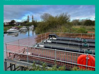
With the ongoing challenges of electrical grid demand, Ebtech advised on a 1,000,000 Litre thermal store to facilitate demand side response. The thermal store provides approximately 1 hour of storage should the business be required to increase or decrease their electrical consumption to balance the grid.
